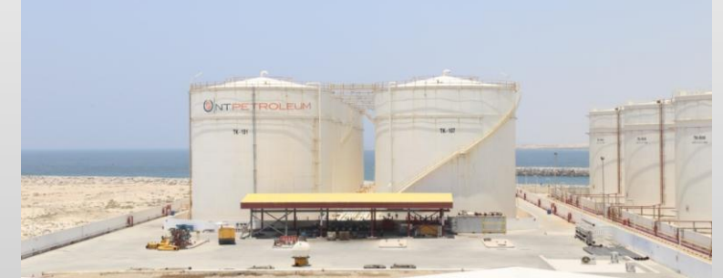
EPC Contractor Oil and Gas Storage Tank Farms
