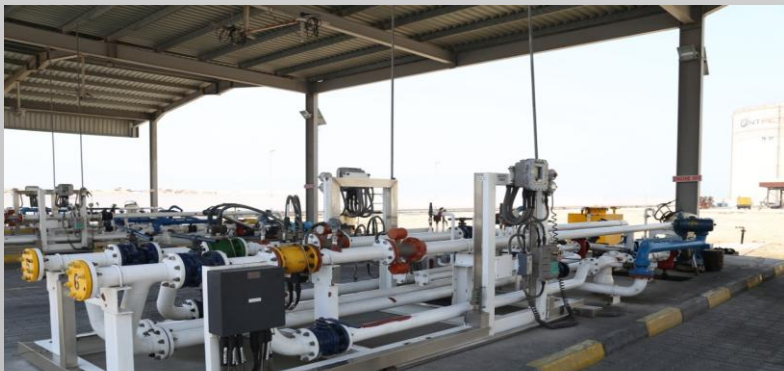
Pump Room Shed Mechanical Works
