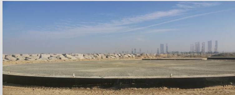
Civil Work Tank Foundation
