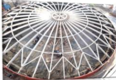
MS DOME ROOF STRUCTURE
