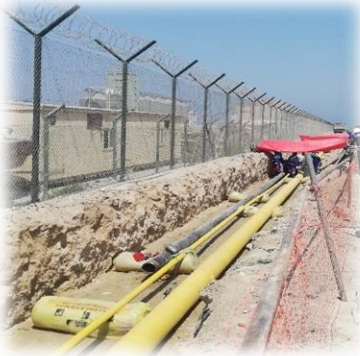
Underground pipeline works
